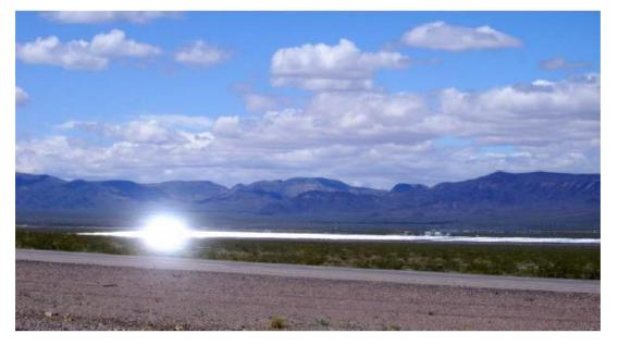
Figure 31 – Picture of a 'glare spot' at a parabolic trough facility in Nevada
